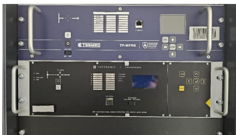
Figure 8-7 EAC relays
